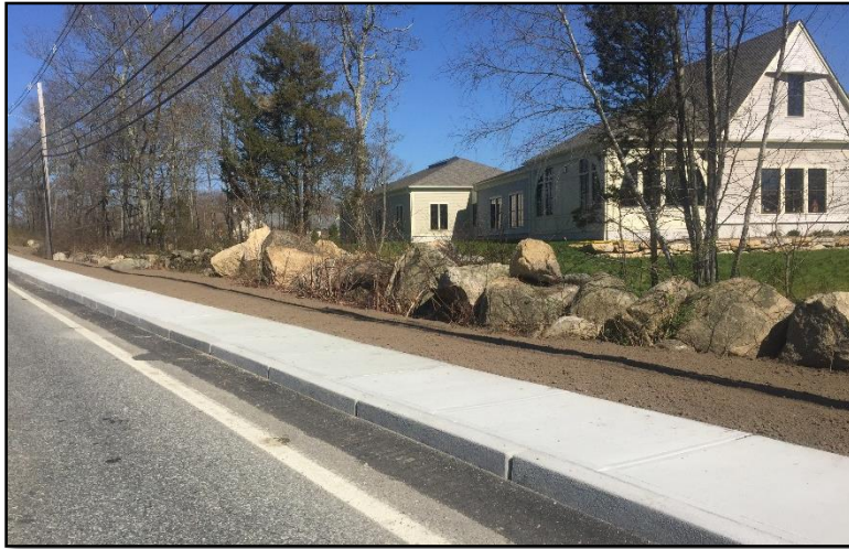
New sidewalk along Bulgarmarsh Road
