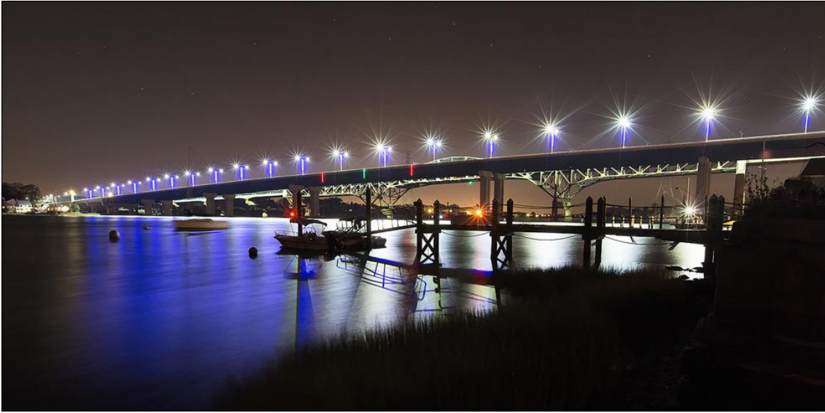
Sakonnet River Bridge
